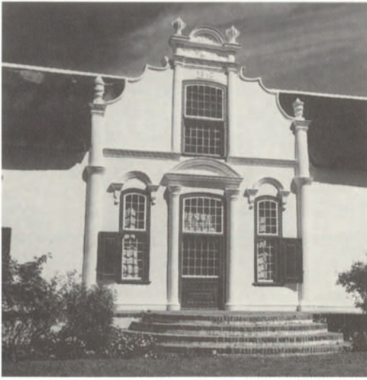
South Africa: Late eighteenth-century country house: Bosch en Dal
