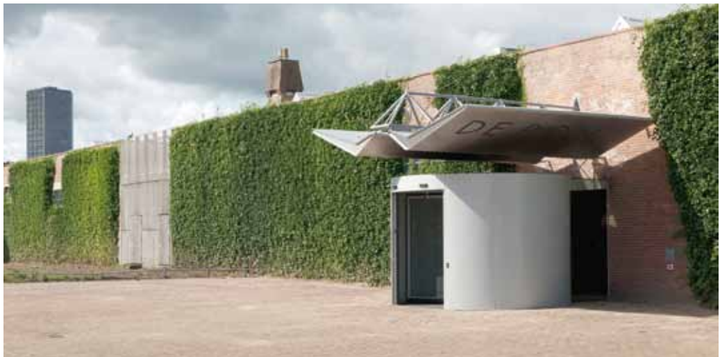
Outside view of Museum De Pont in Tilburg © Peter Cox.
