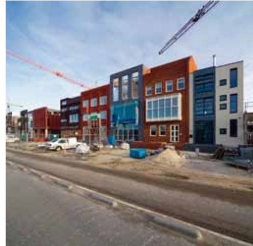
A new road under construction © Pi de Bruijn – de Architecten Cie.
