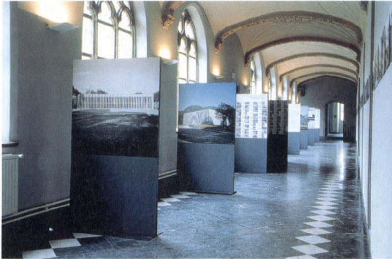
A former Dominican monastery became a school of architecture in Ghent. The restoration was carried out in several stages under the direction of architect Herman de Witte and finished in 2001. Photo by Marc Dubois.
